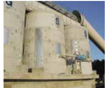
Concrete mix plant Sand silo
